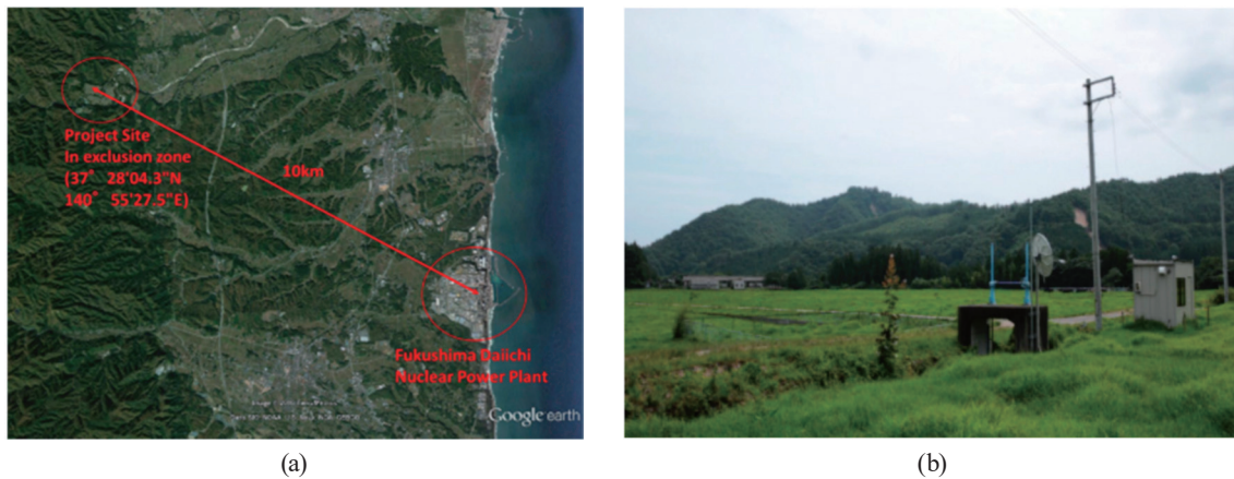
Fig. 10. (Color online) (a) Project site in the Fukushima exclusion zone (37° 28' 4.3\" N, 140° 55' 27.5\" E; 10 km from Fukushima Daiichi Nuclear Power Plant) and (b) sink node station. (7)
