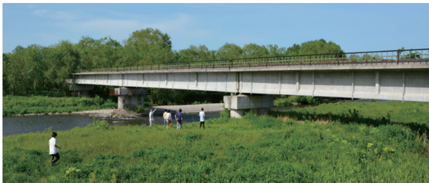
Fig. 4. (Color online) General view of Mukagawa Bridge.
