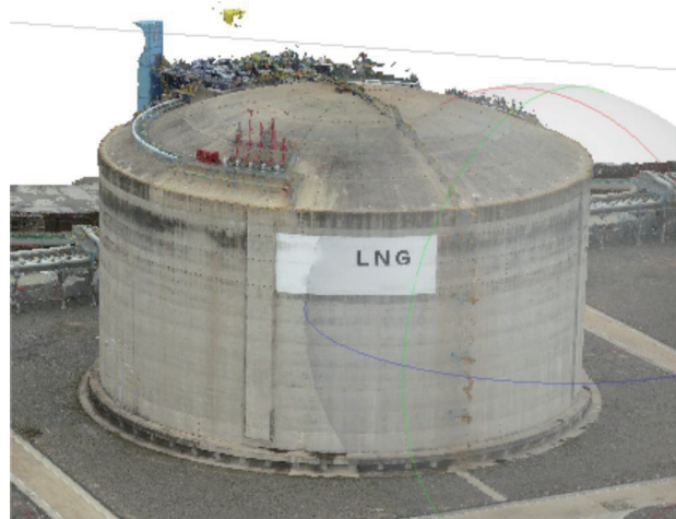
Fig. 2. (Color online) The target LNG storage tank of the study.
