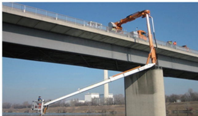
Fig. 1. (Color online) Close inspection using bridge inspection vehicle.
