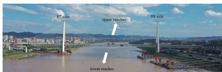
Fig. 4. (Color online) Yangtze River Bridge of Baijusi in Chongqing.
